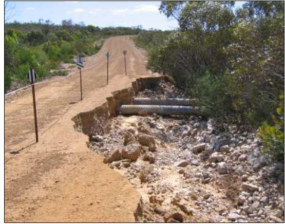
Road damage caused by heavy rain
