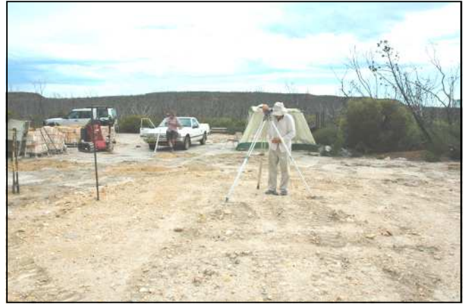
Ric Pepper surveys levels for the new Twertup building.
