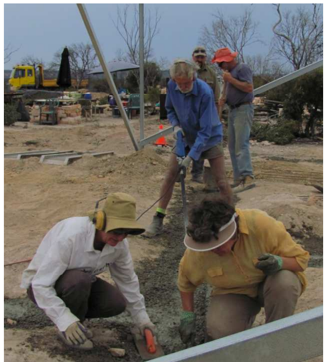
There was no gender bias on this work site, Gil and Geraldine trowel off the footings, Bill spread the concrete and Ric checks all is OK. Photo J. Thompson
