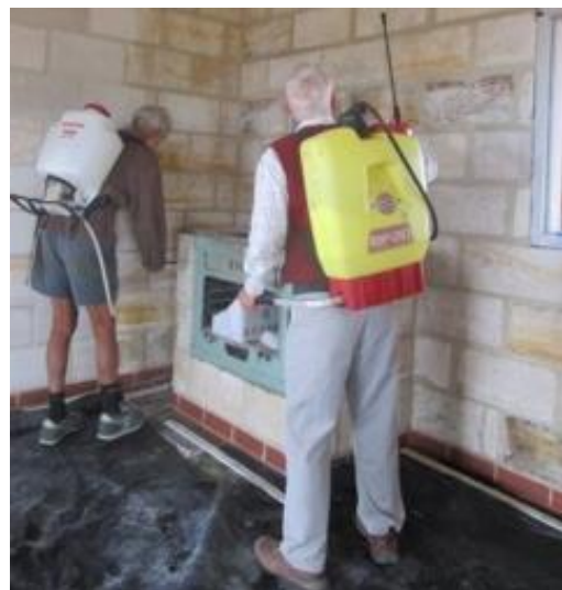
Bill Thompson and Ron Richards spray sealant on the interior walls.
